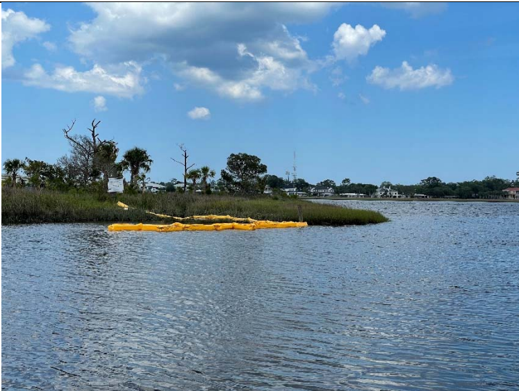
Photo 6: New turbidity barrier and manatee signs.
