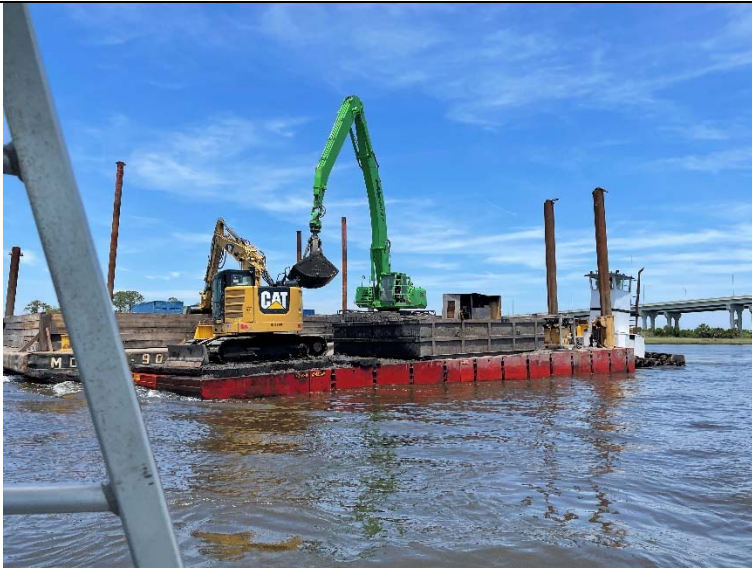
Photo 5: View of Barge setup in the intracoastal and active material removal from smaller, 20' wide barge at the time of the inspection.
