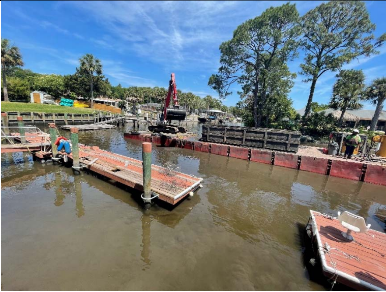
Photo 1: 20' Wide Barge actively dredging within Baseline 2.
