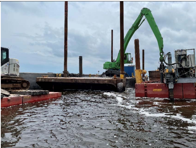
Photo 2: View of 26' Thruster Barge actively off-loading before returning to Baseline 1.
