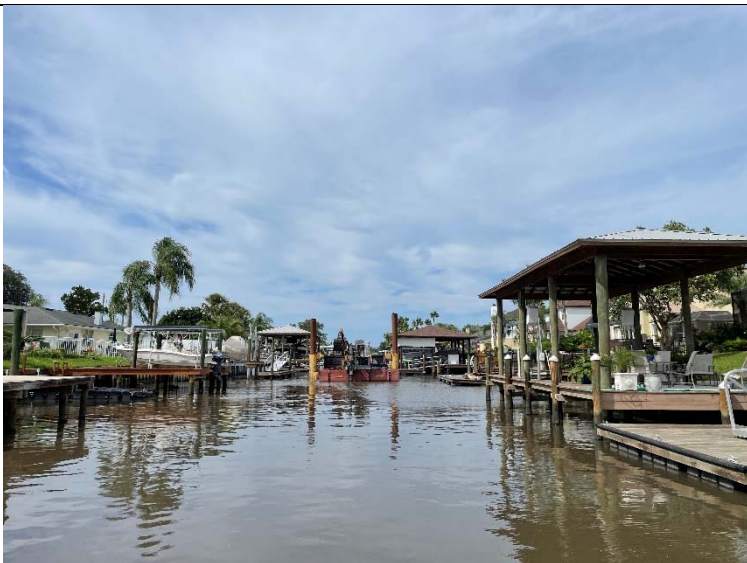
Photo 2: View of 26' Thruster Barge located in Baseline 5: Southern IOP.
